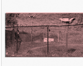
Fencing at Gold Base showing motion-activated lights
